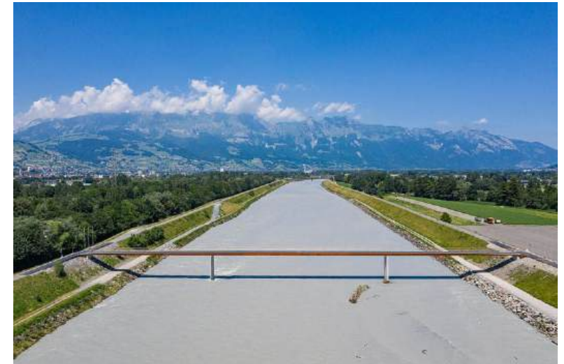
Buchs-Vaduz cycle and pedestrian bridge. Source: Agglomeration Werdenberg-Liechtenstein
