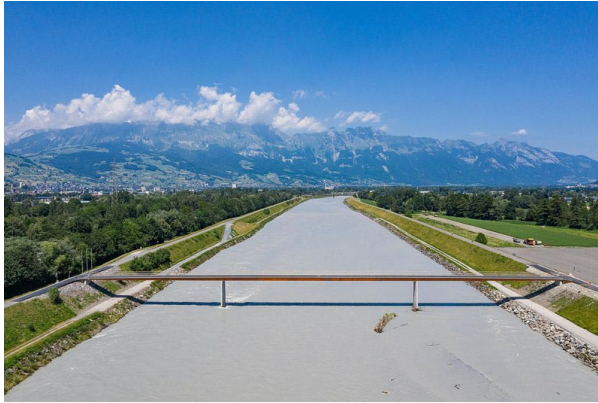
Buchs-Vaduz cycle and pedestrian bridge. Source: Agglomeration Werdenberg-Liechtenstein
