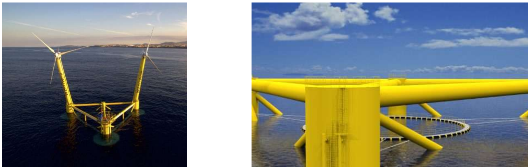
Figure 1 W2Power floating technology with space for aquaculture
