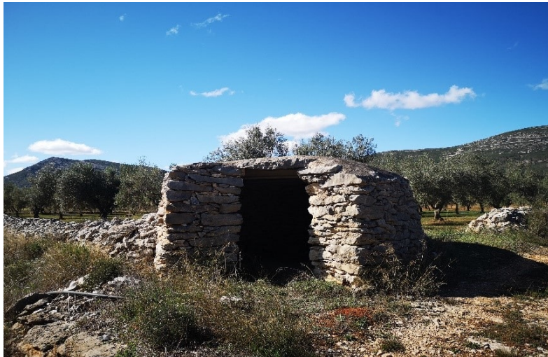
Figure A4.5: Pedra en sec (dry stone), traditional construction technique in the Alt Maestrat An ancient pastoral refuge
